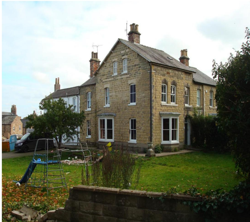
Fig 2. View of Front (west) Side (north) Elevation. Site of new proposed Hot Tib and New French Doors to bay window centre section.
