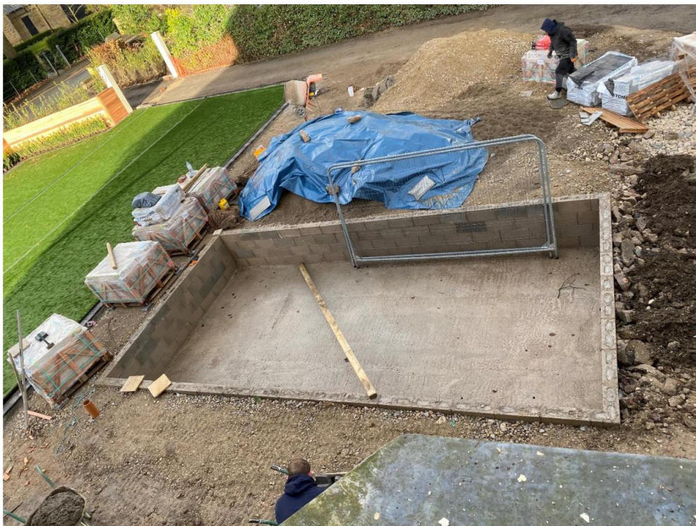
Fig 5 Pocket position for the Hot Tub already constructed.
