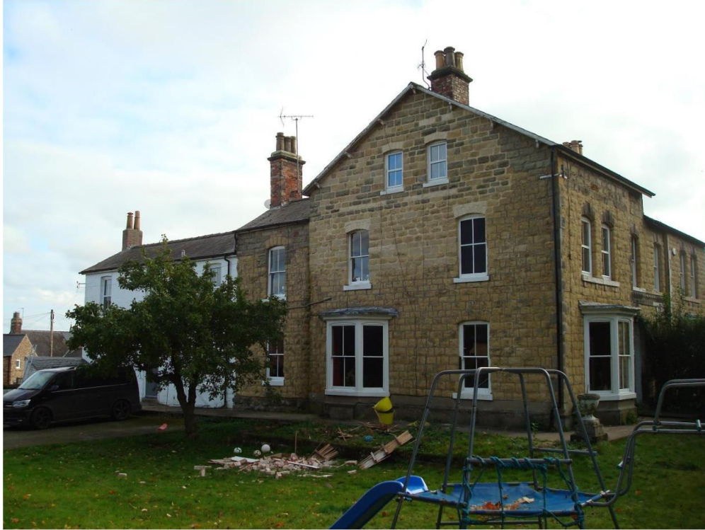
Fig 3. View of Side (north) Elevation. Site of new proposed French doors replacing centre window of bay.
